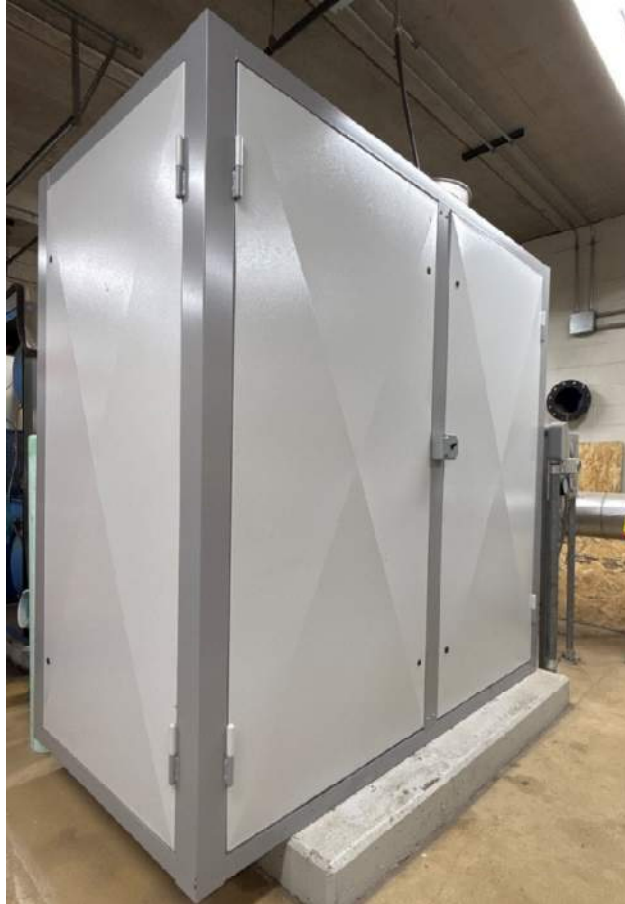
Figure 5-14: Screw Blower Enclosure
