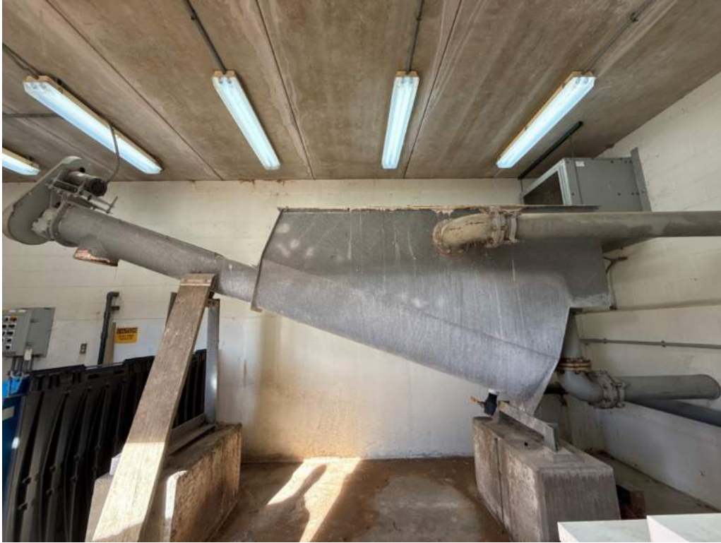
Figure 5-6: Grit Classifier and Washer
