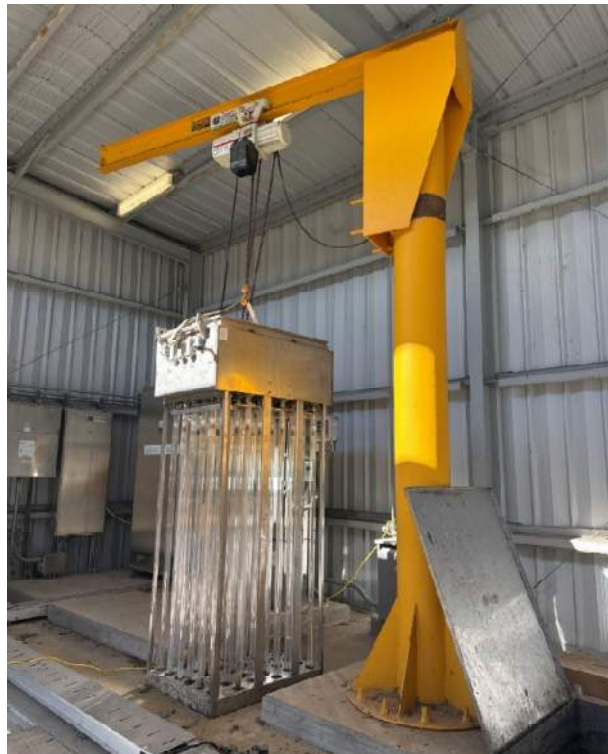
Figure 5-17: UV Disinfection Channel and Bulbs
