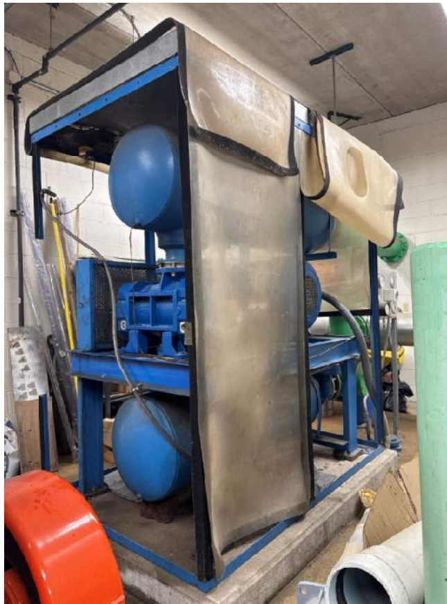
Figure 5-13: Positive Displacement Blower
