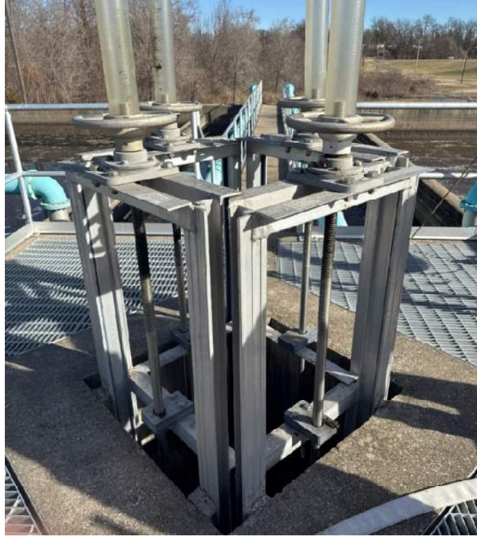
Figure 5-11: SBR Splitter Structure Manual Gates
