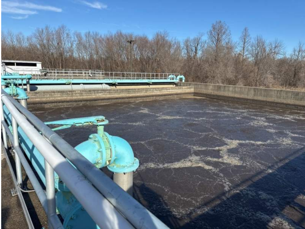
Figure 5-9: SBR Basin During Aeration Cycle
