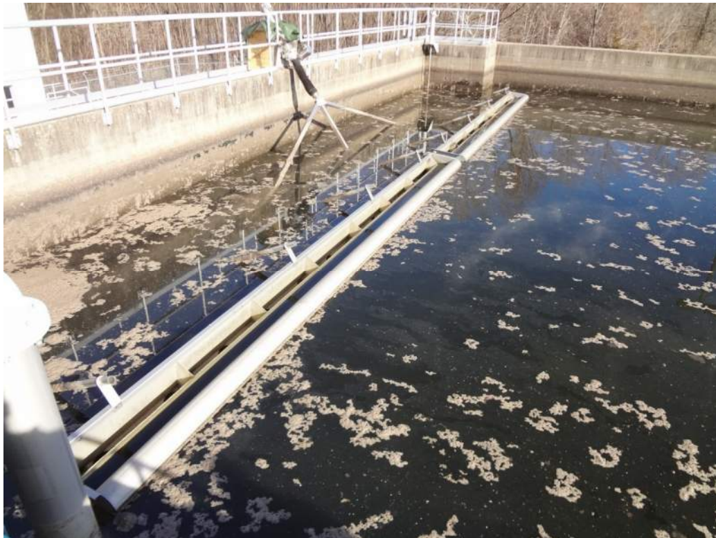
Figure 5-9: SBR Basin During Aeration Cycle
