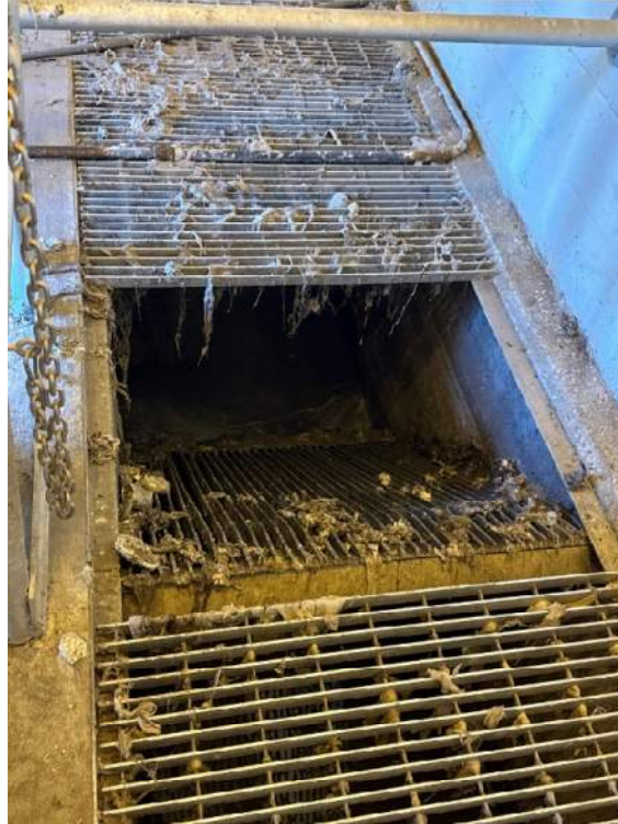
Figure 5-3: Manual Bypass Screen
