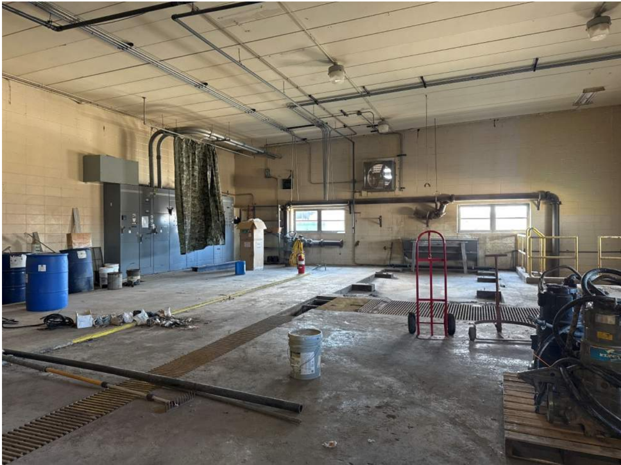
Figure 5-20: Future Dewatering Equipment Area
