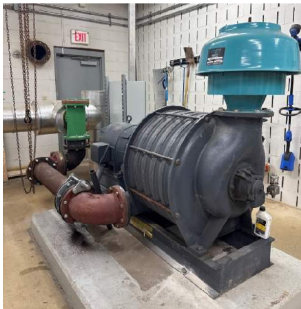
Figure 5-14: Screw Blower Enclosure
