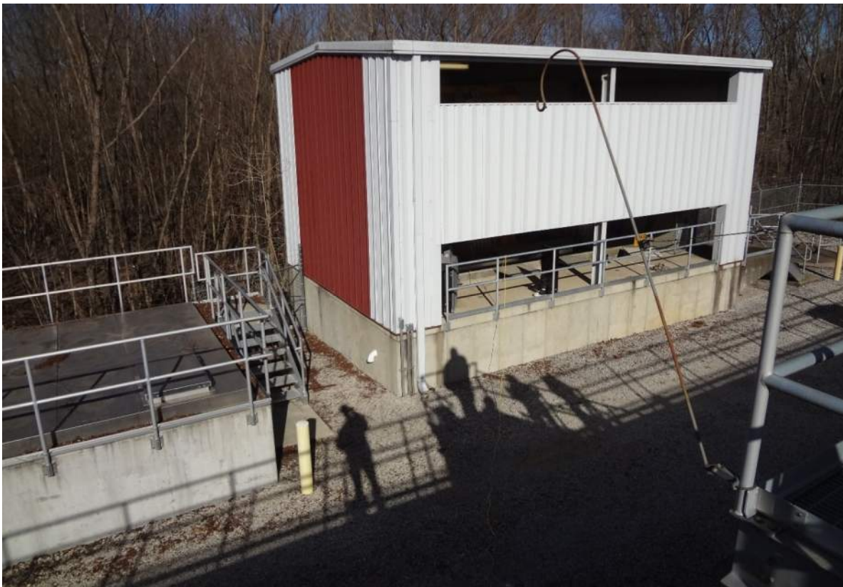
Figure 5-16: UV Building and Finger Weir Structure
